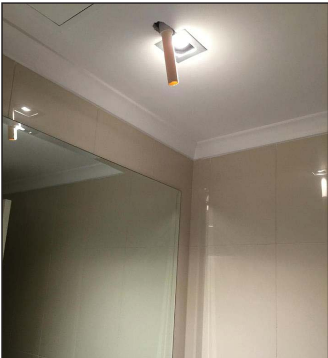
Pipe through bedroom ceiling taking water to bathroom sink
