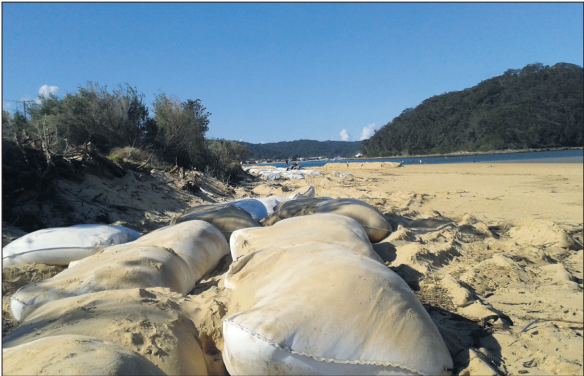
The sandbag wall along The Esplanade at Ettalong may be replaced by other revetment work
