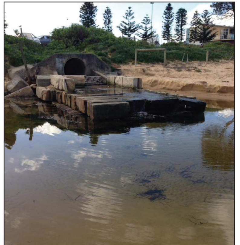
Storm water scour in front of the main outlet near the surf club
