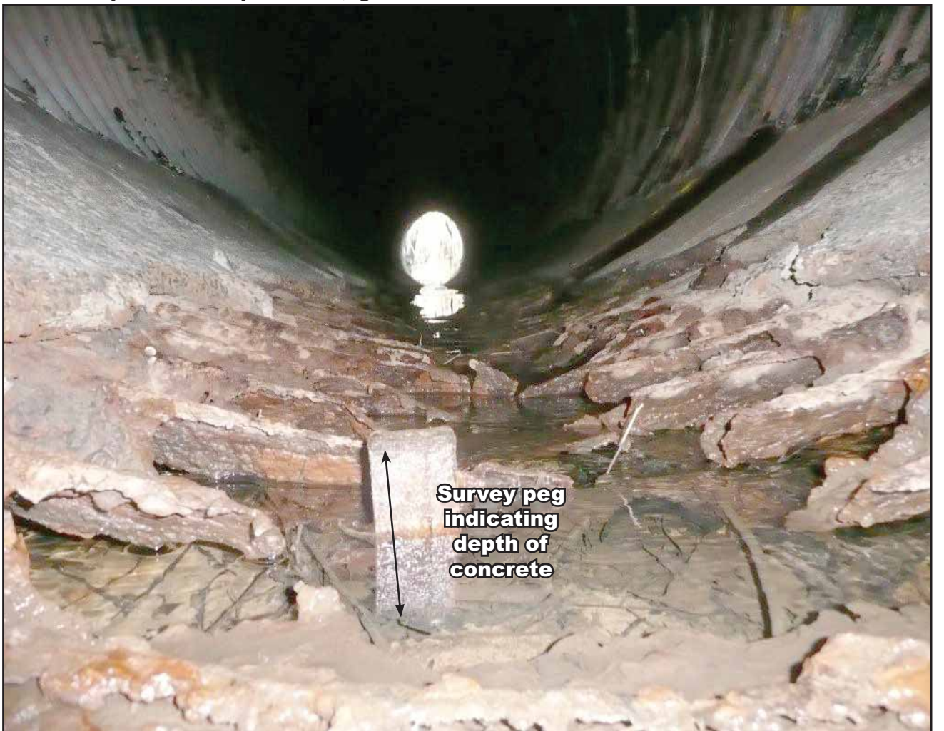
This photograph shows evidence concrete was used not once but twice in two pipes located in the upper reaches of Mooney Mooney Creek beneath Peats Ridge Road
