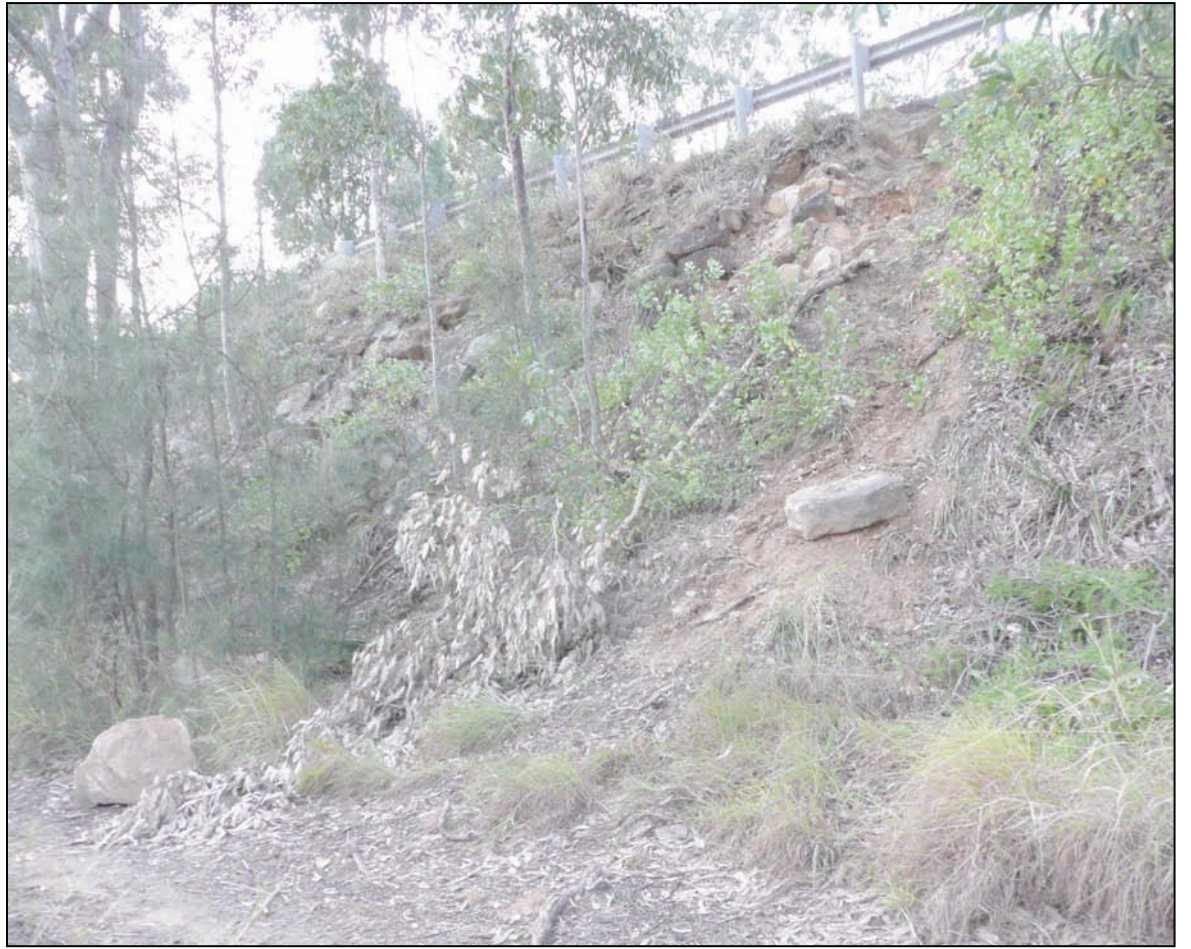
The embankment below Mt Ettalong Rd near the hairpin bend at the eastern end of Patonga Dr where rocks and a tree debris have fallen down onto the dirt track below.
