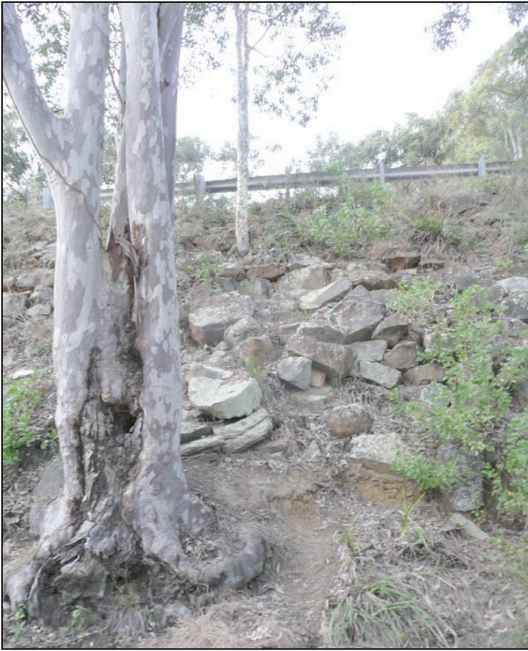
The embankment below Mt Ettalong Rd near the hairpin bend at the eastern end of Patonga Dr where rocks and a tree debris have fallen down onto the dirt track below.
