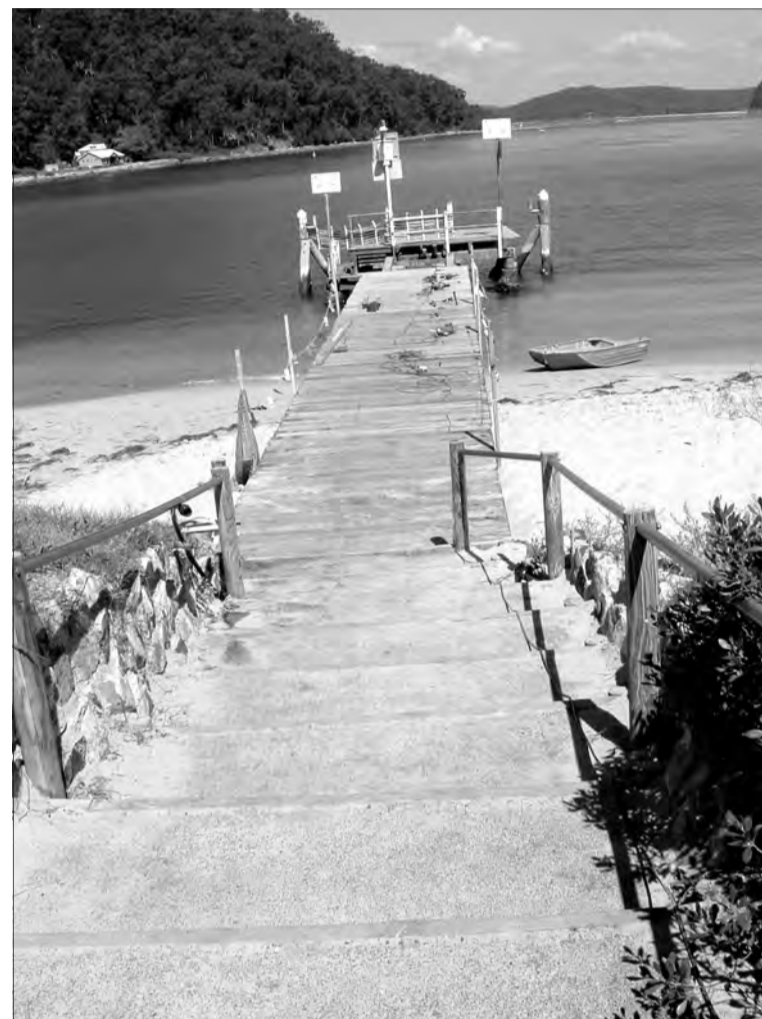
Ferry Street Wharf
