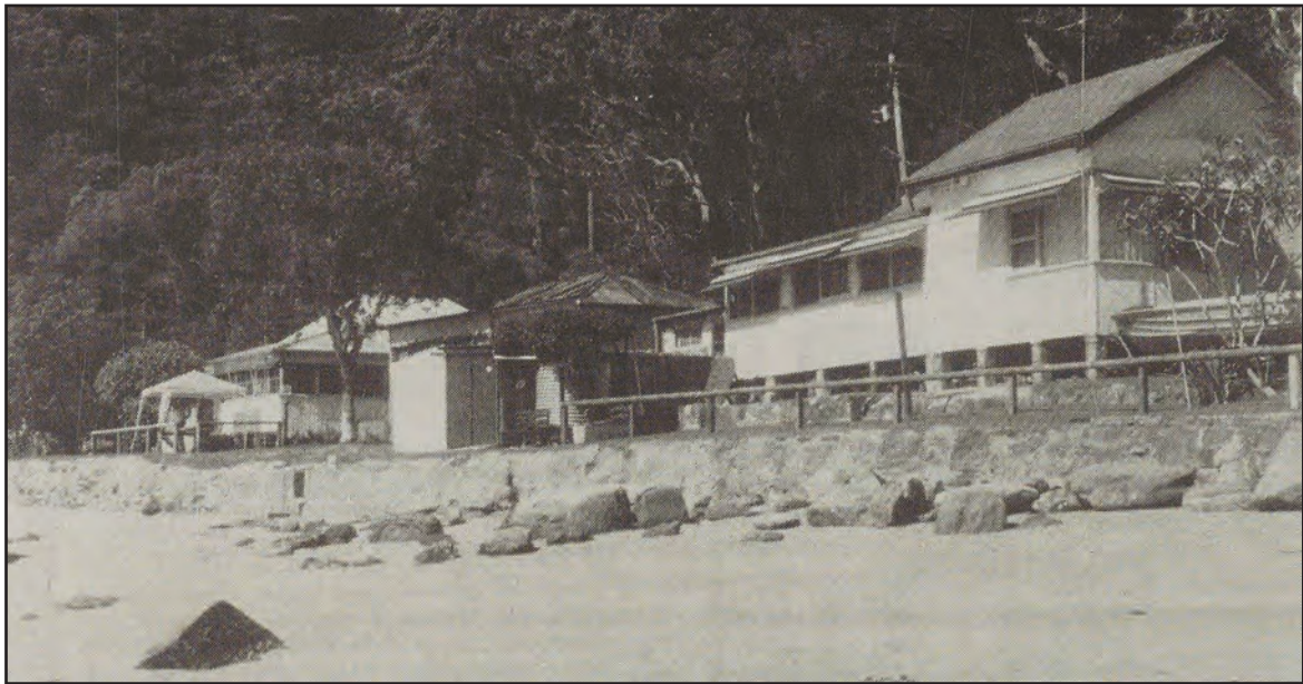
Heritage buildings at Dark Corner
