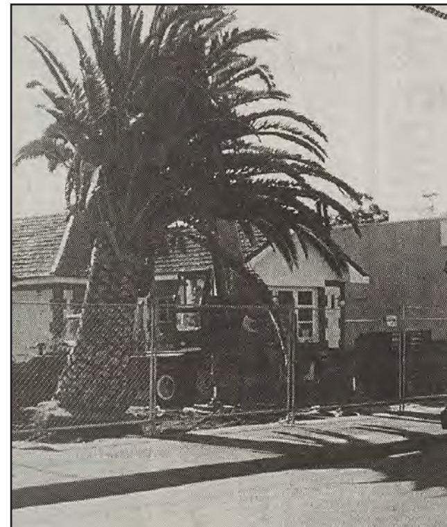
A giant palm tree being lowered into position
