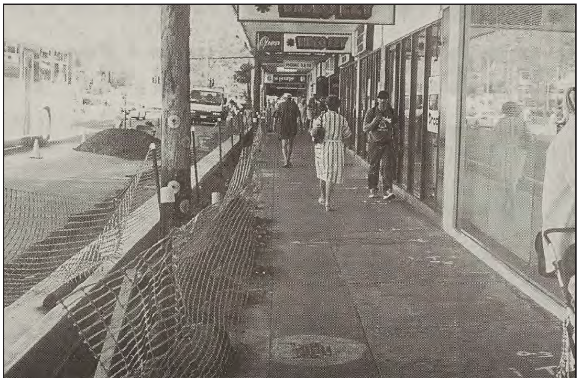
The partially completed Woy Woy footpath upgrade viewed heading towards the railway station
