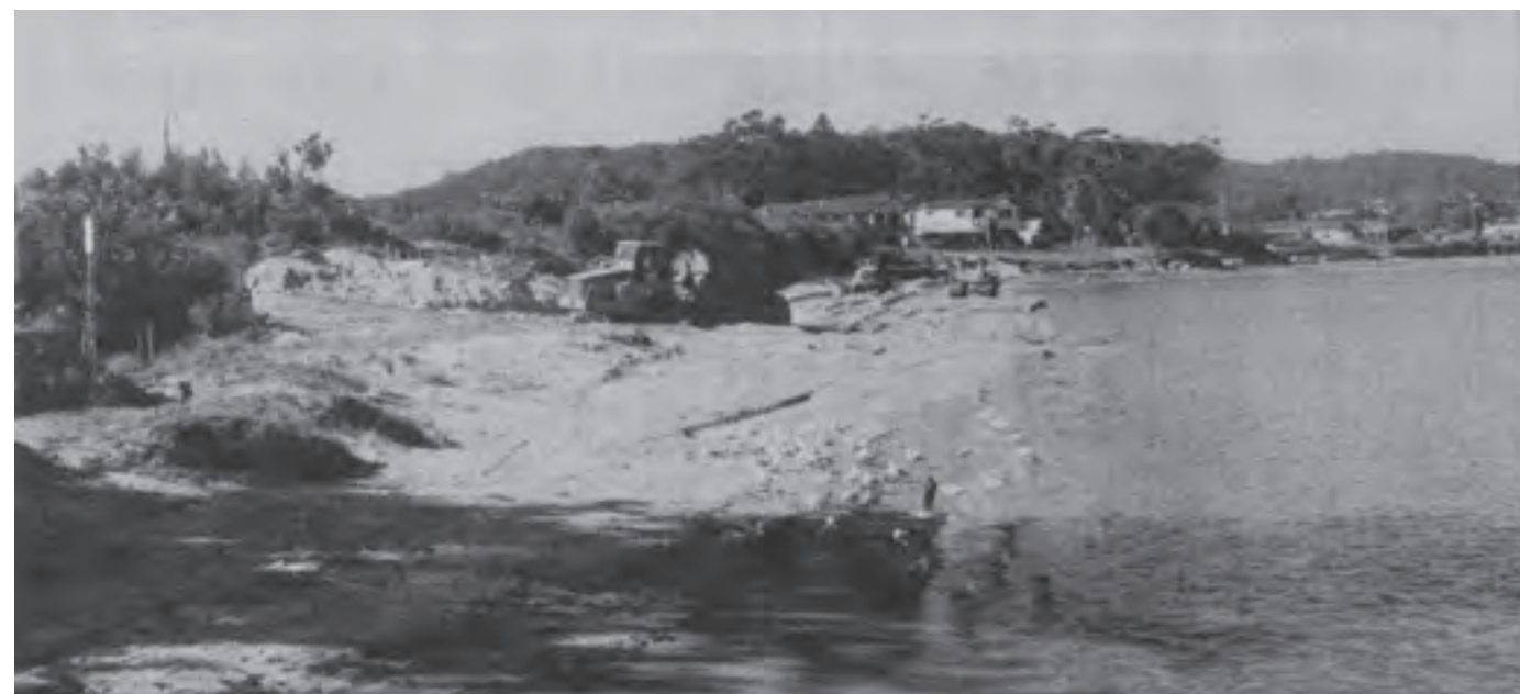
Dump truck hauling some of the 15,000 cubic metres of sand used as part of Ettalong Beach's renourishment facelift
