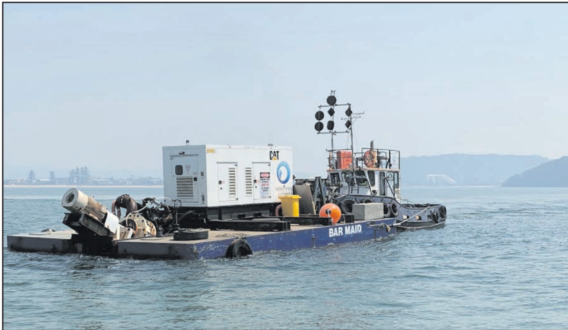
The dredge at Ettalong Channel
