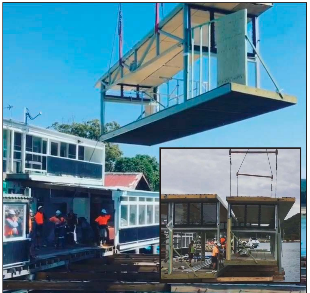
Prefabricated extensions were lowered into place at Fishermen's Wharf Woy Woy
