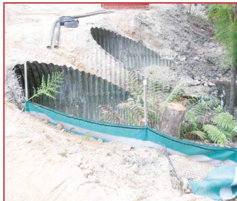
The two pipes shown in these three photos ran under Peats Ridge Road and were lined with concrete when put in place almost thirty five years ago. Both eight foot diameter culvert pipes had their concrete linings repaired at least once during their years of good service. The NSW Coroner was, during the inquiry into the deaths of five people in Piles Creek Somersby, misled when Gosford City Council allowed the court to understand that Council had no knowledge or experience in the use or application of concrete to protect the structural integrity of corrugated steel culvert pipes which it was expected to maintain. Council is on public record in the Express Advocate advising readers that they, Council inspect all roads and structures twice each year. The pipes have been removed during recent months and all traces of the existence of concrete lined steel culvert pipes has been completely buried
