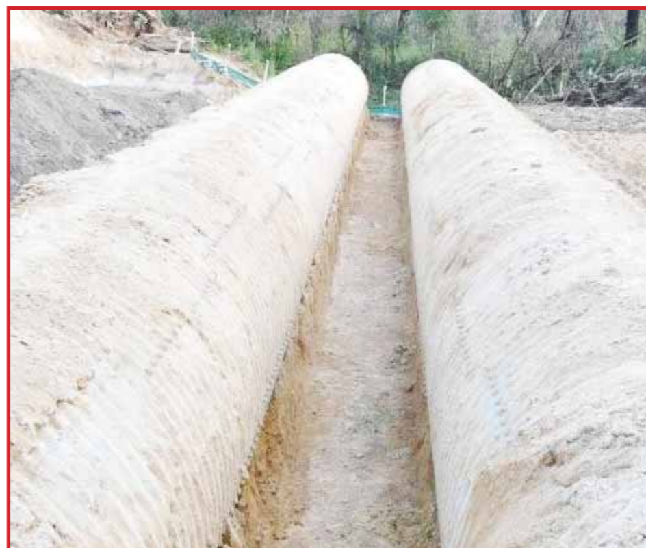
The two pipes shown in these three photos ran under Peats Ridge Road and were lined with concrete when put in place almost thirty five years ago. Both eight foot diameter culvert pipes had their concrete linings repaired at least once during their years of good service. The NSW Coroner was, during the inquiry into the deaths of five people in Piles Creek Somersby, misled when Gosford City Council allowed the court to understand that Council had no knowledge or experience in the use or application of concrete to protect the structural integrity of corrugated steel culvert pipes which it was expected to maintain. Council is on public record in the Express Advocate advising readers that they, Council inspect all roads and structures twice each year. The pipes have been removed during recent months and all traces of the existence of concrete lined steel culvert pipes has been completely buried
