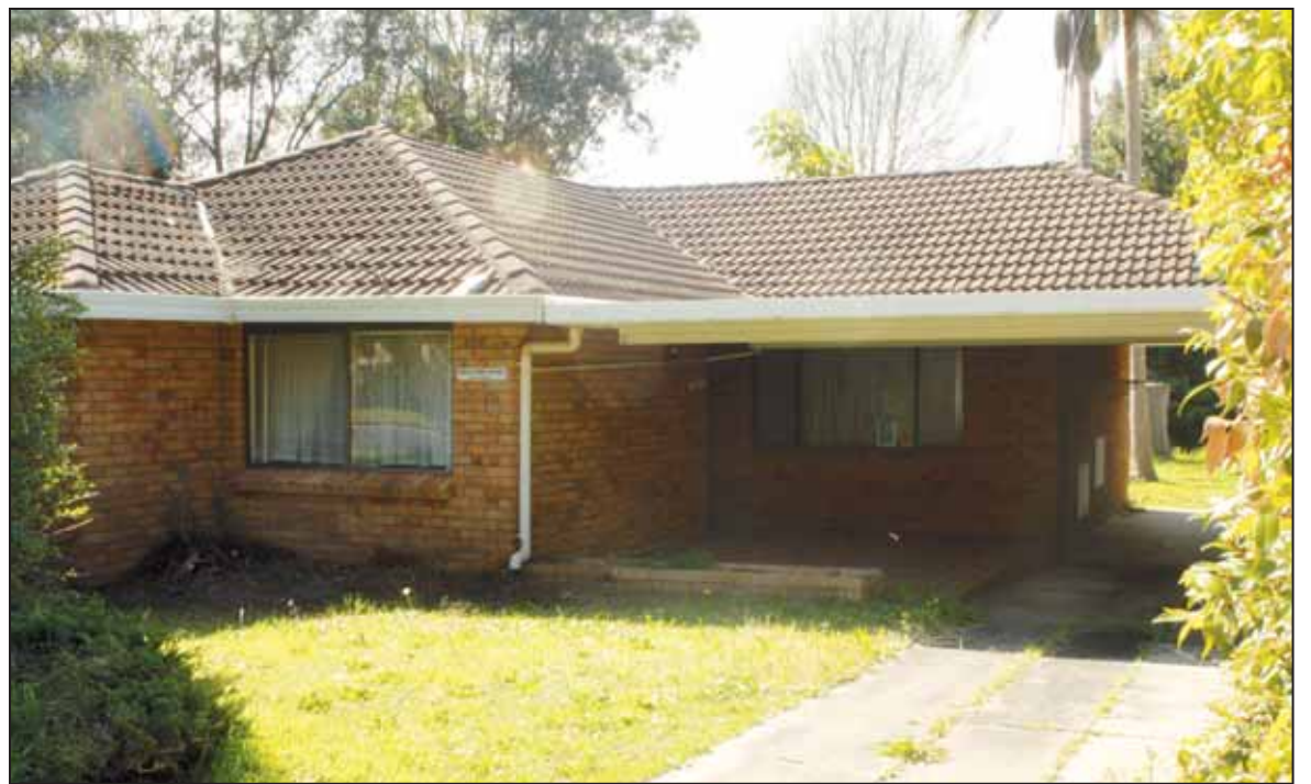
The house to be demolished on Neera Rd, Umina
