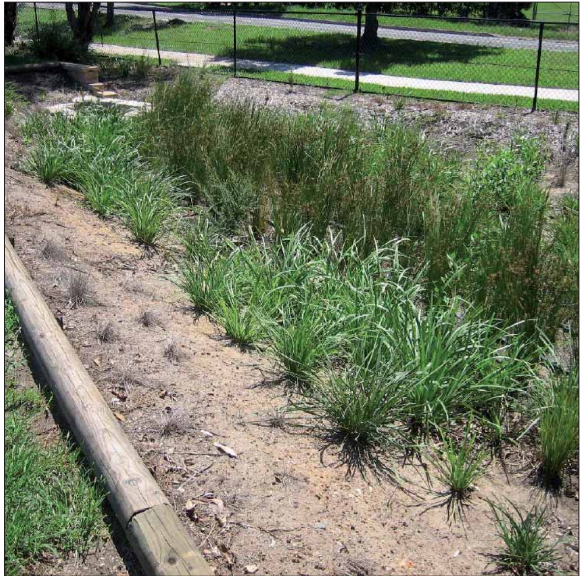
Sediment trap as part of a stormwater treatment train
