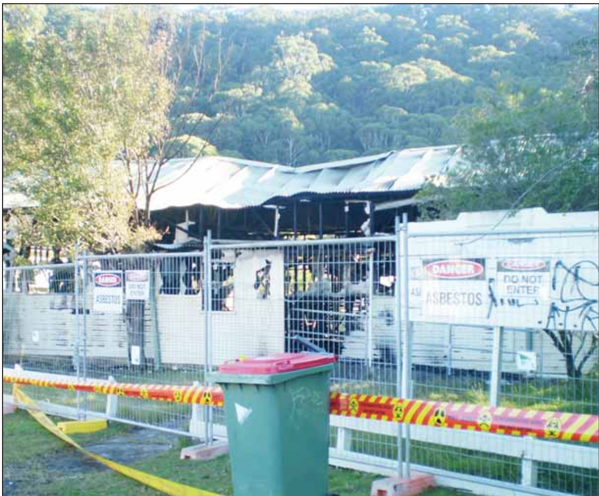
The remains of Ettalong Progress Hall
