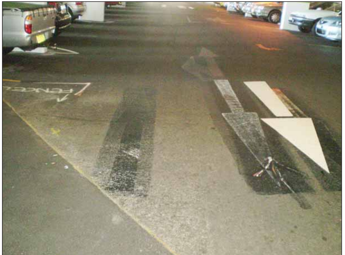
Arrows repainted at Woy Woy commuter car park
