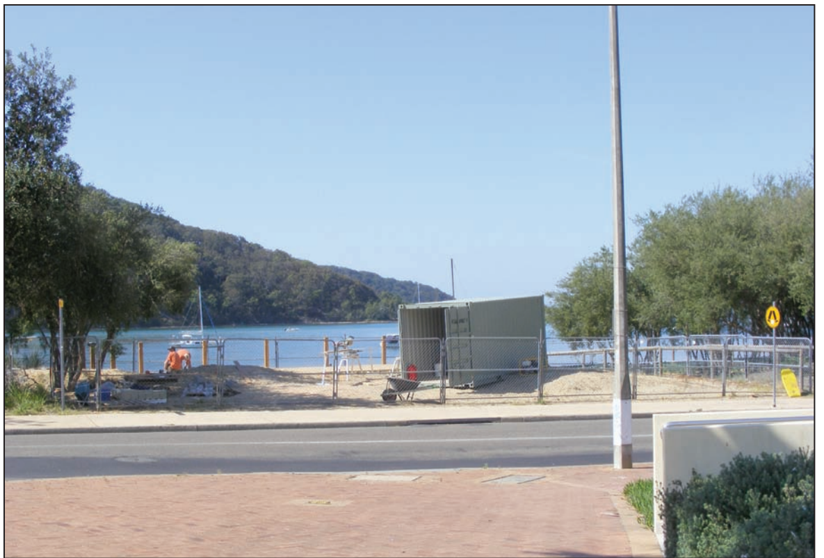
Ettalong Foreshore viewing platform work commences
