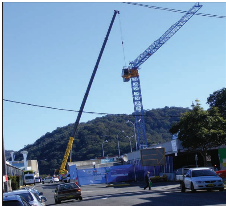
Expansion work continues on the Woy Woy Commuter Carpark
