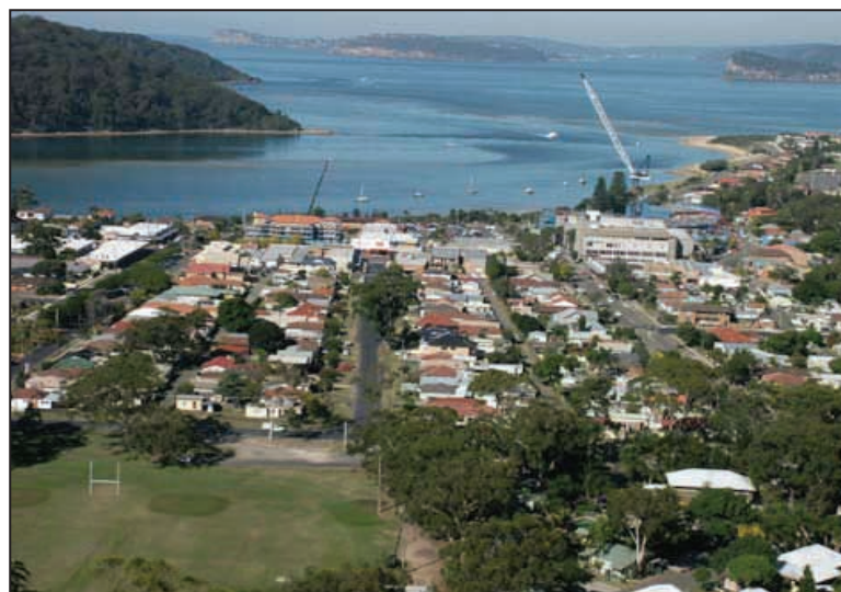
Overlooking the entrance to Brisbane Water where dredging works are expected to take place before Christmas (photo source: Gosford Council)
