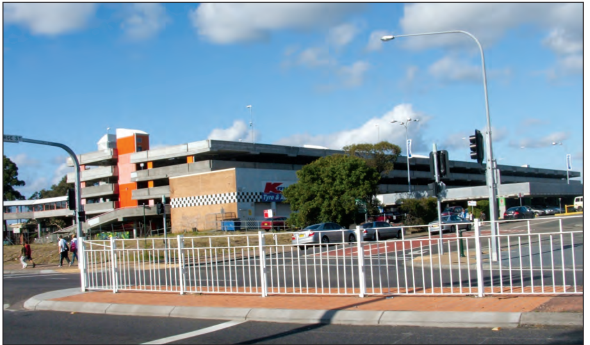
The multi-level Woy Woy Commuter Car Park
