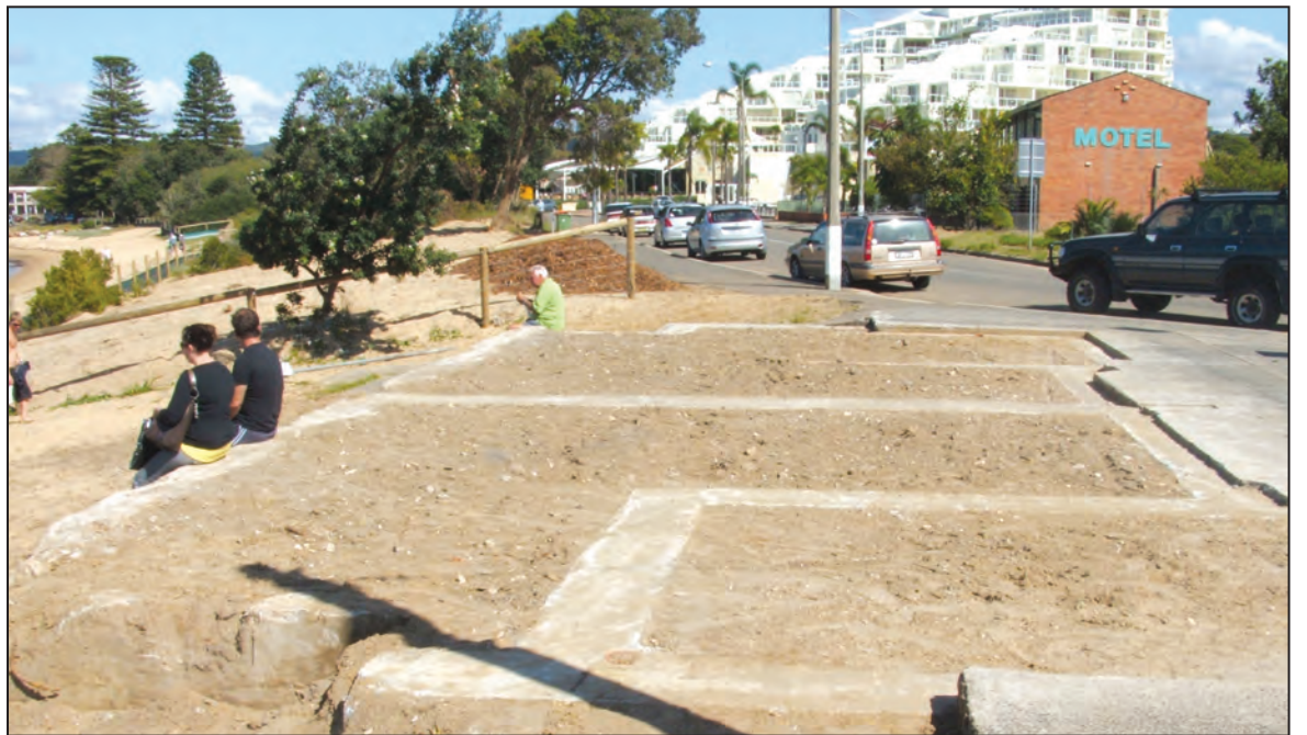
The site of the demolished toilets on the Ettalong Foreshore
