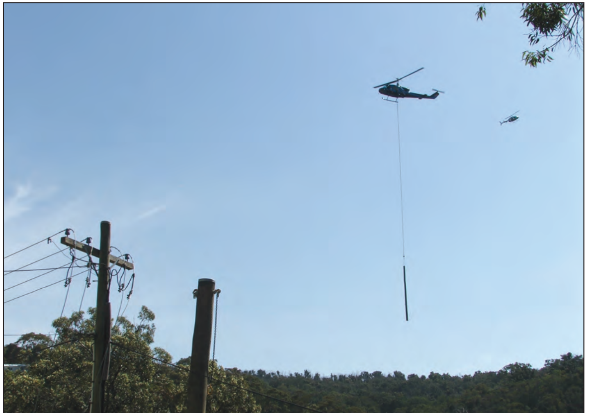
Poles being transported to Horsfield Bay via helicopter
