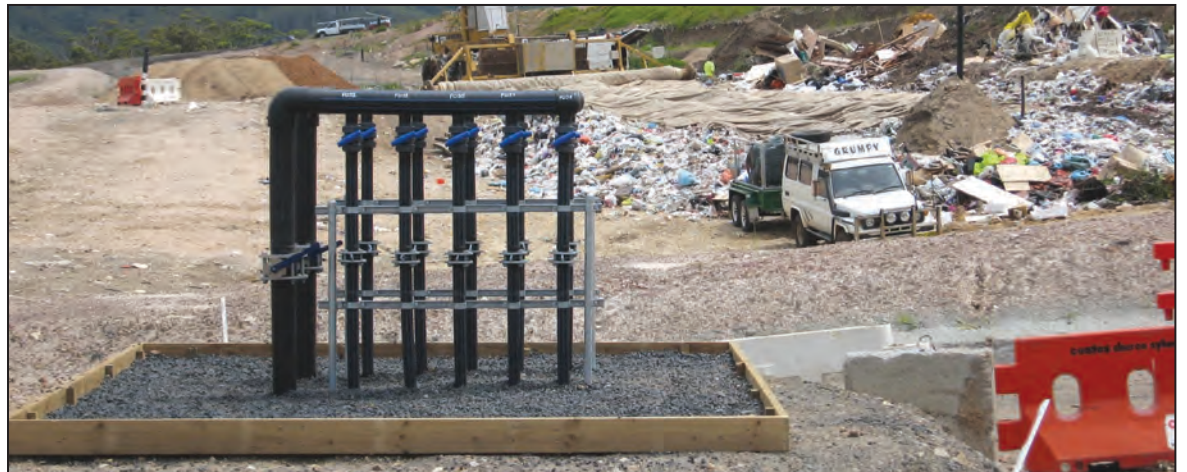
A gas well installed at the Kincumber Tip
