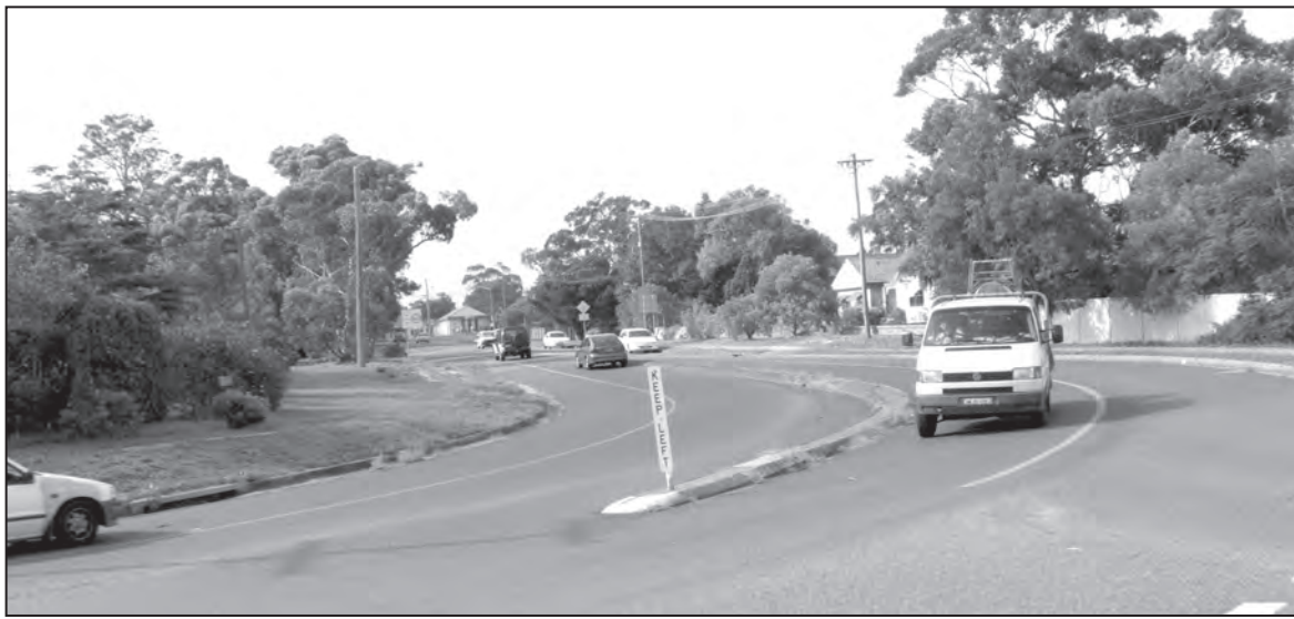
Sydney Avenue between Hobart Ave and Brisbane Ave
