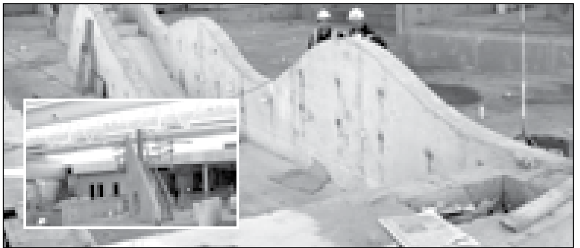
Water slides under construction at the leisure centre
