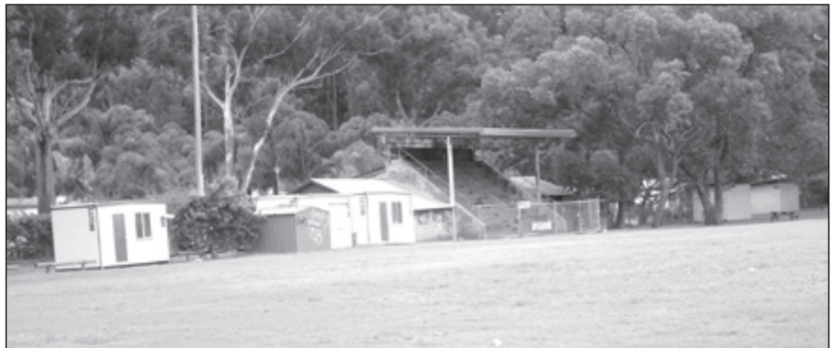
The grand stand at Ettalong Oval, surrounded by security fencing after a recent fire
