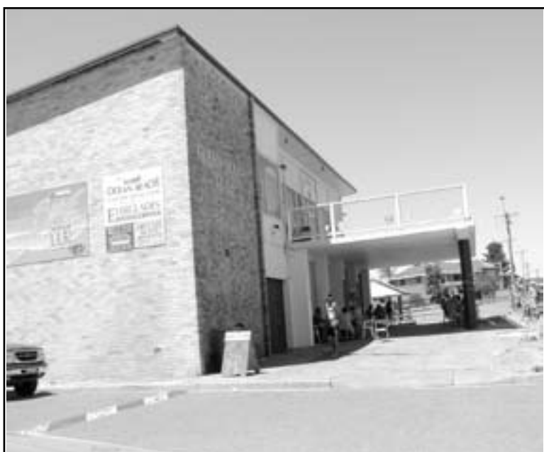
Ocean Beach Surf Club soon to be renovated
