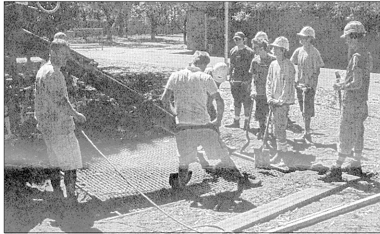
HSC Construction students from BWSC Woy Woy Campus
