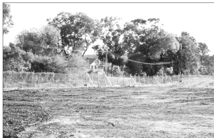
Cleared site for the Peninsula Leisure Centre
