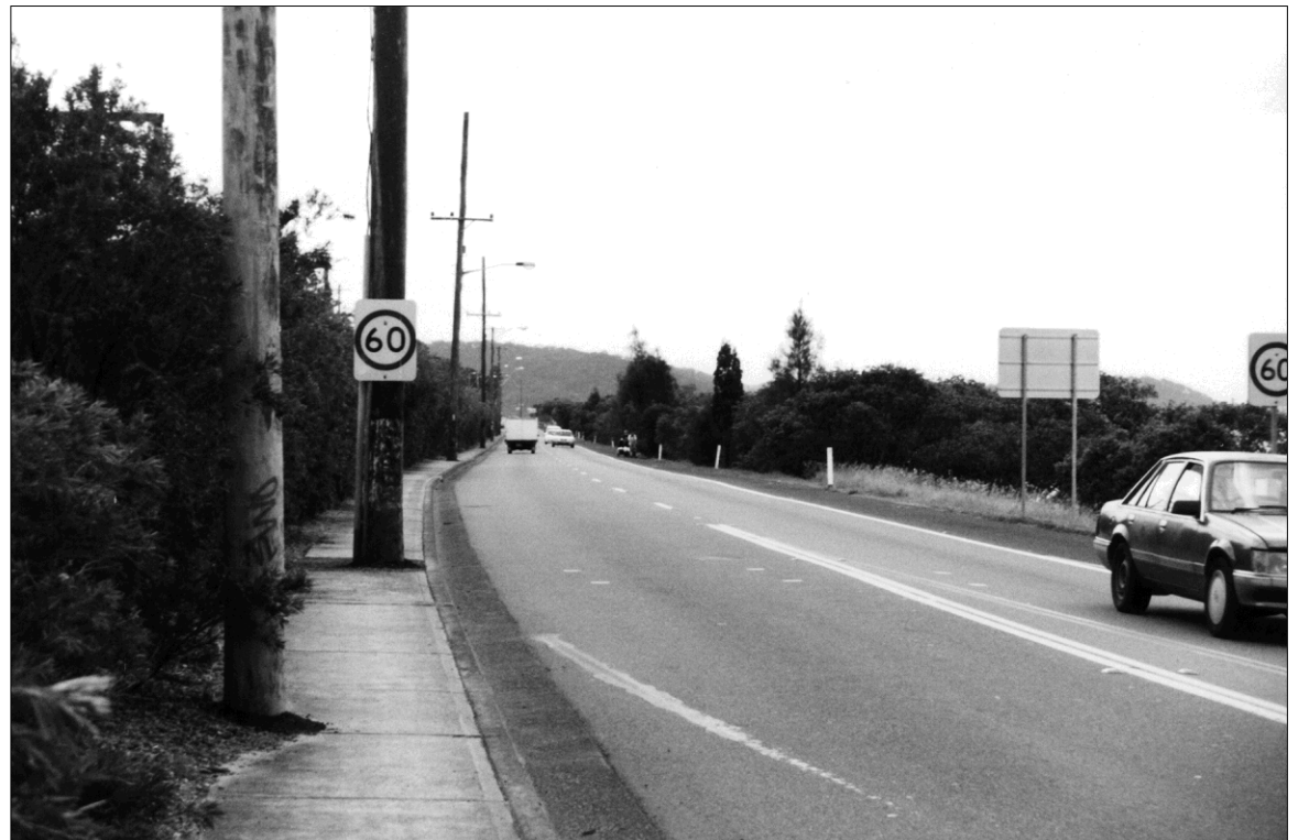
Construction of the Koolewong to Woy Woy section of cycleway will begin next year
