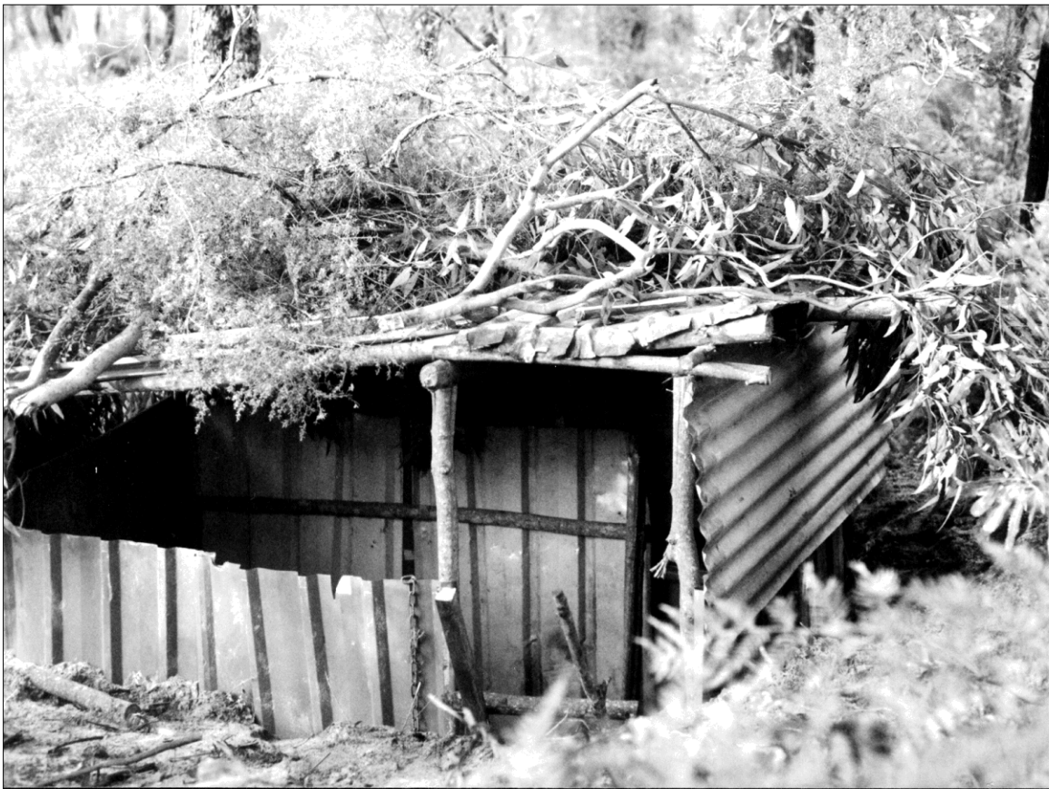
Burrawang Bushland Reserve was damaged with the construction of this illegal hut
