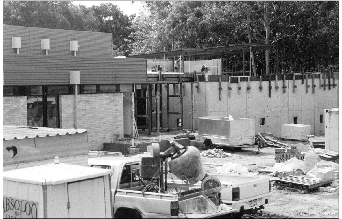
Construction continues at the Woy Woy Local/Children's court
