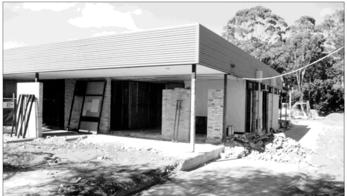
Work underway at Woy Woy courthouse
