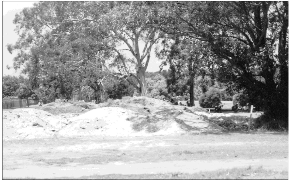
Mounds of earth on the golf course in preparation for proposed earth works
