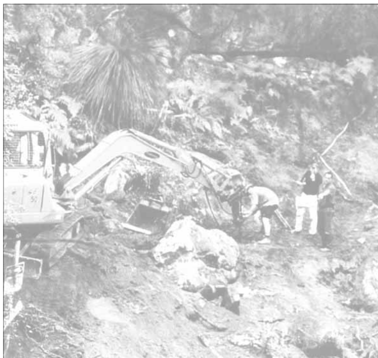
Clearing under way at Woy Woy Bay
